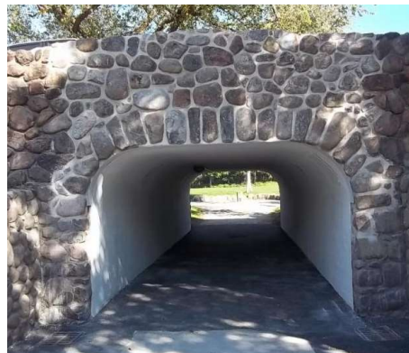
Stockton Drive Underpass, 1926
